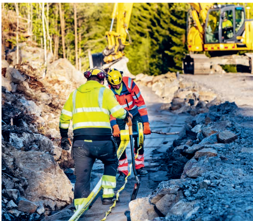
Construction of the Ribäckens wind farm in Finland. Photo: Joachim Lagercrantz
