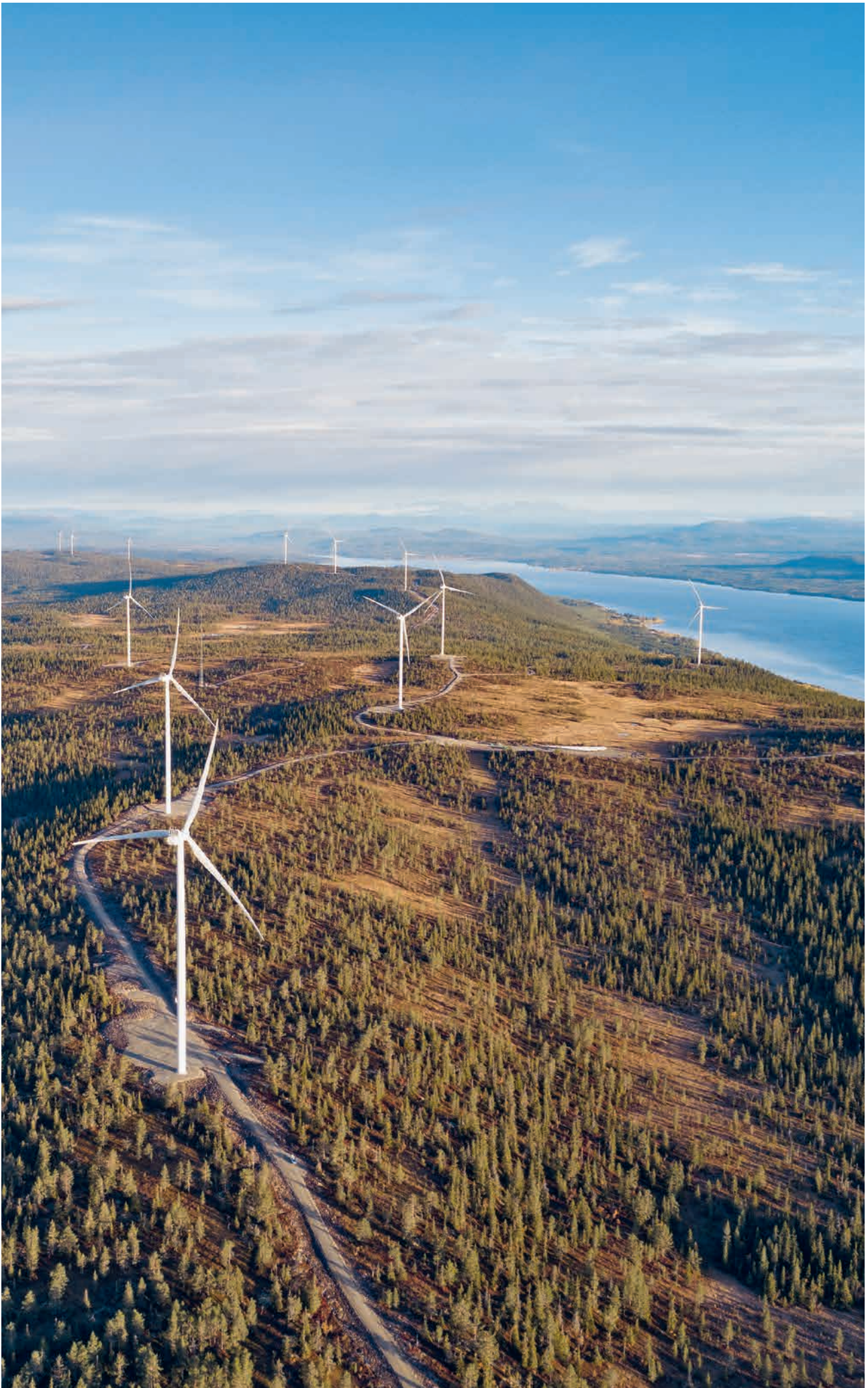
The Raskiftet wind farm (112 MW) in Norway. Photo: Joachim Lagercrantz
