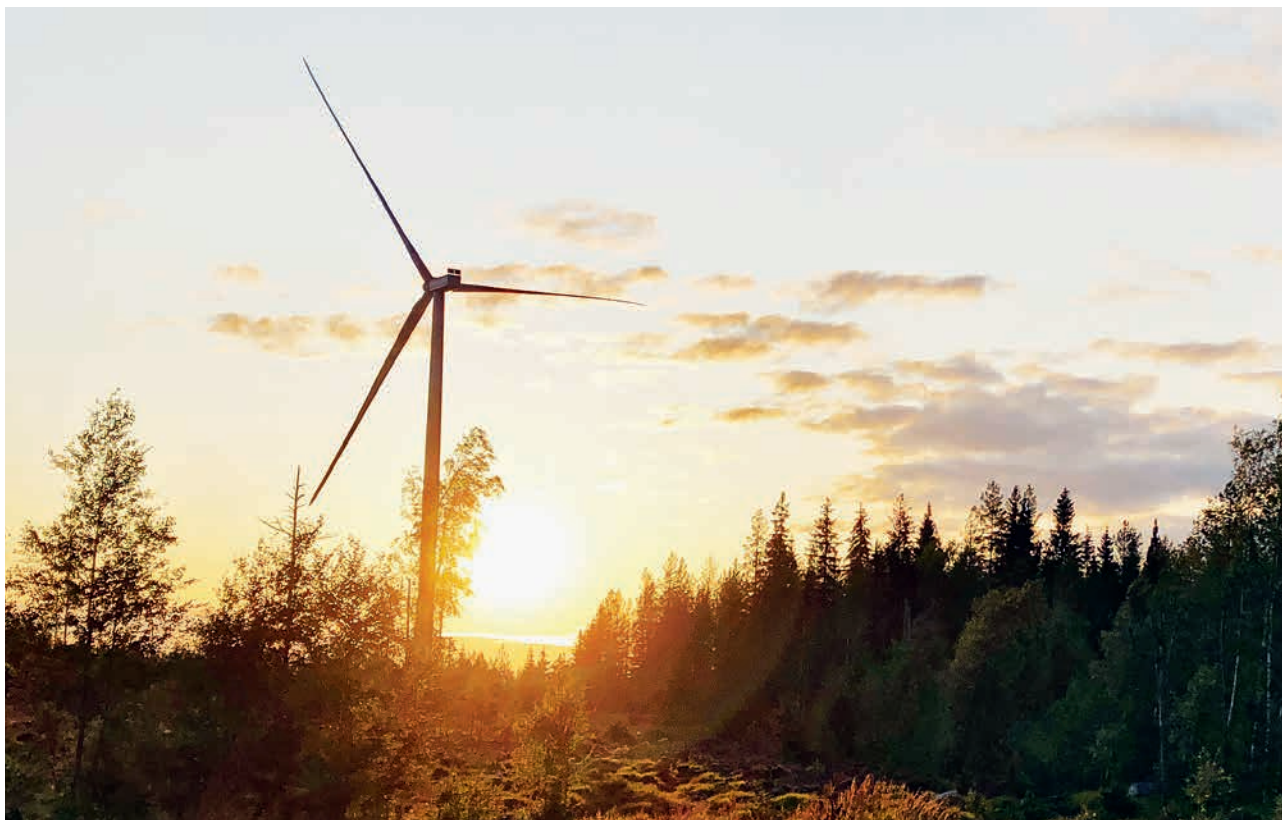
The Ponsivuori wind farm (30 MW) in Finland was commissioned and handed over to IKEA. Photo: Matti Latva-Hirvelä/Carelin
